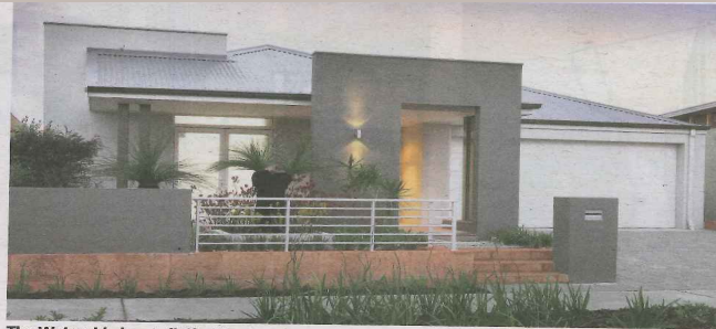
The Waterside has a distinctive, contemporary-style facade.
